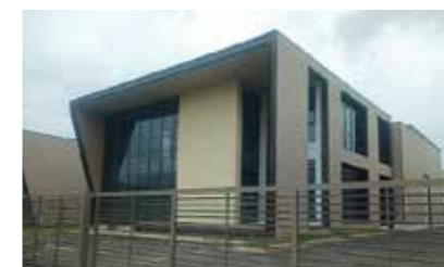
HSP PLANT E, SABAH (In Construction)
